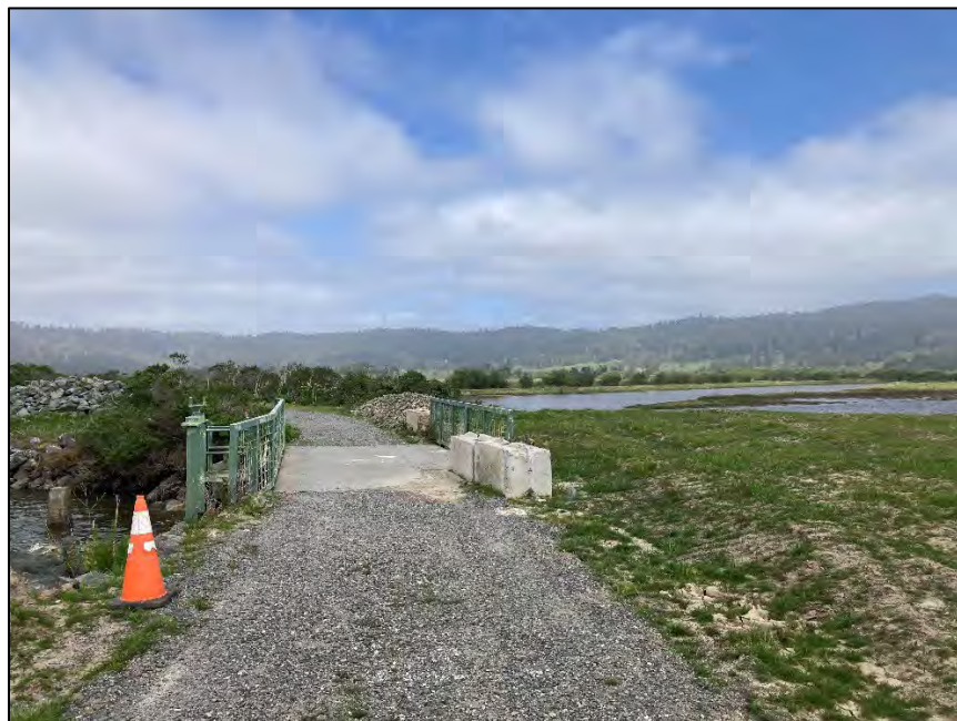
Photo 8: Top view of Long Pond tide-gate structure, with backfill on right and entrance to Hookton Slough to the left. Tide-gates are currently chained shut.
