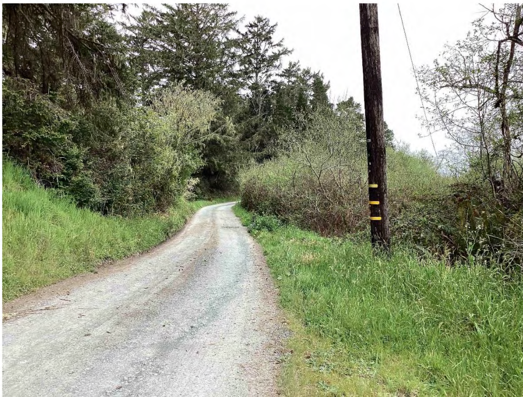
Photo 13—View of another low point in Refuge Access Road that will be raised to prevent flooding, looking south.
