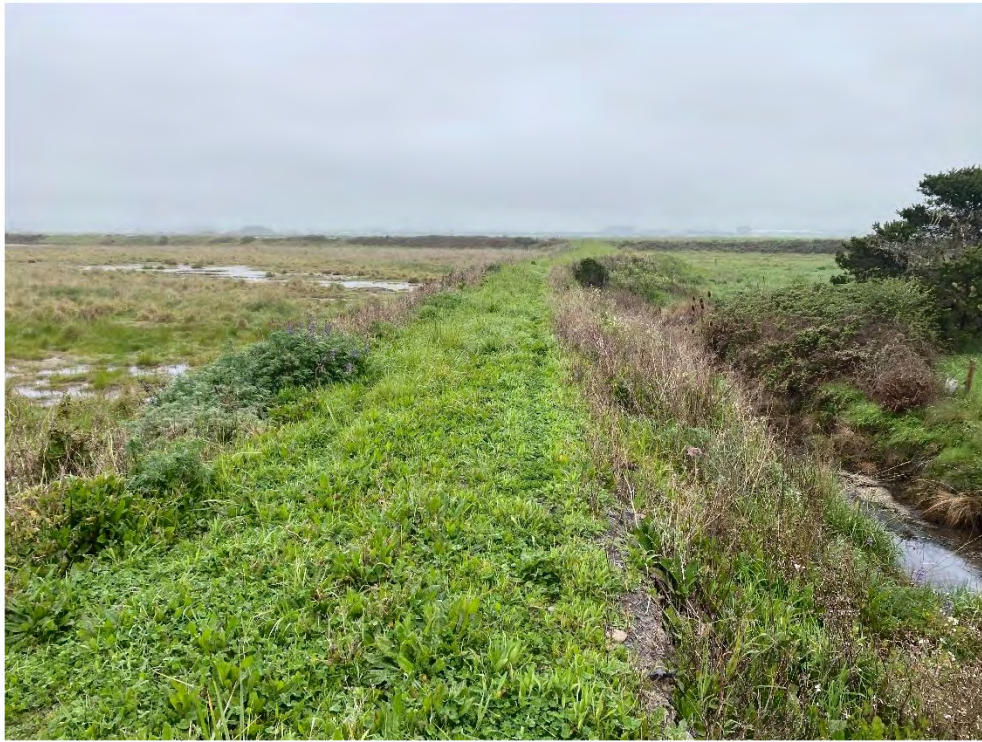
Photo 1—Southern cross levee in its current condition, looking east toward Mad River Slough levee. The cross levee was constructed circa 2019 when the Mad River Slough levee breached and the adjacent property flooded to the south (picture right). The Project Area still receives intermittent brackish water intrusion from the impaired Mad River Slough levee.
