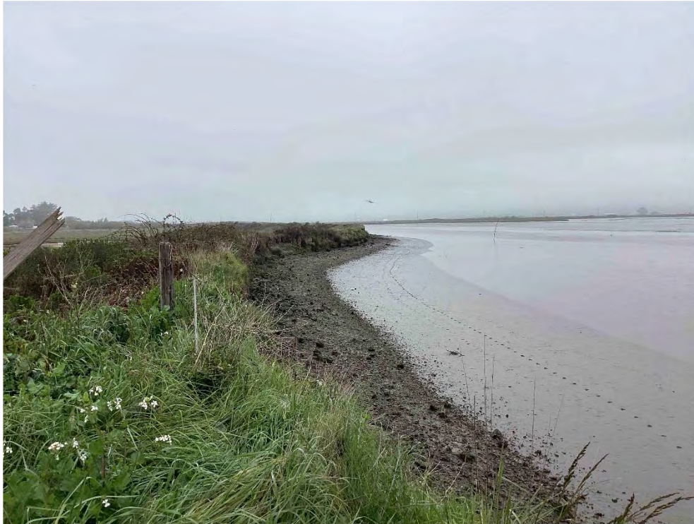
Photo 3—At the eastern-most extent of the southern cross levee, looking north at the Mad River Slough Levee. The levee is variable in height along its length due to scour, which has compromised its longevity and has allowed for salt water to seep to the west of it.
