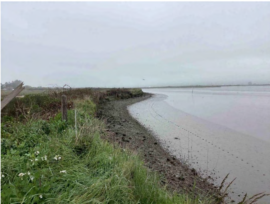
Photo 7: At the eastern-most extent of the southern cross levee, looking north at the Mad River Slough Levee. The levee is variable in height along its length due to scour, which has compromised its longevity and has allowed for salt water to seep into the Project Area.
