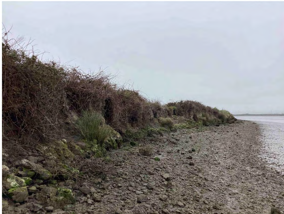
Photo 4—Outboard edge (east) of Mad River Slough levee, where the breach has occurred (the “saddle” seen in the background), and location of the failing tide gate (out of frame). Portions of the levee will be lowered during Project construction to allow tidal waters to flow into the Project Area. Portions of the levee are expected to become salt marsh.
