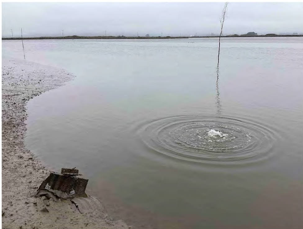
Photo 5—The tide gate “bubbling” as ponding water from the west of the levee drains. The tide gate will be removed in the final stages of Project construction to complete the levee breach and allow the Mad River Slough to infiltrate into the Project Area uninhibited, and restore a natural tidal regime.
