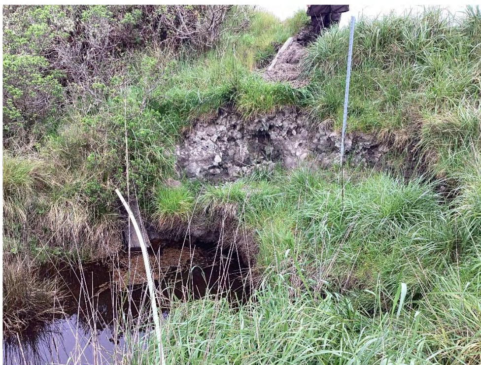
Photo 6—Inboard edge (west) of the Mad River Slough levee, where the interior drains through the tide gate. This area will be excavated to form a subtidal to permanently flooded channel that supports eelgrass, and is the main “entrance” for tidal waters to feed the rest of the lagoon channel system.
