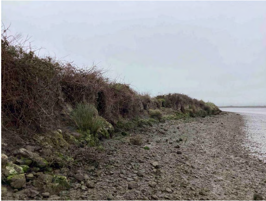
Photo 3: Outboard edge (east) of Mad River Slough levee, where the breach has occurred (the "saddle" seen in the background), and location of the failing tide gate (out of frame).
