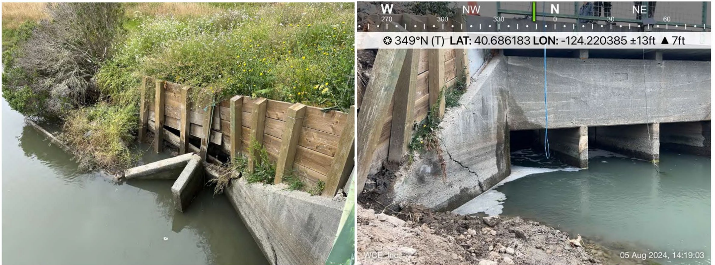
Figure 3: Damage to South Wingwall of the Long Pond Tidal Gate
